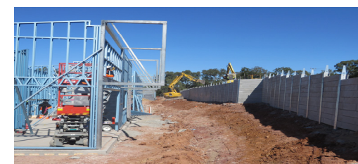
ERECTION OF WALL FRAMES AND RETAINING WALL BELOW GENERAL PARKING.
