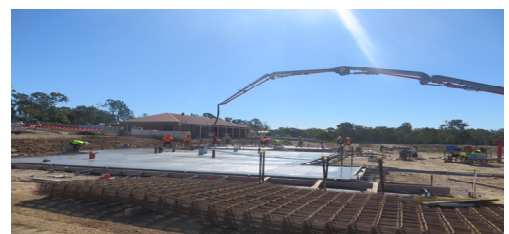
CONCRETE SLAB TO CANTEEN COMPLETED
