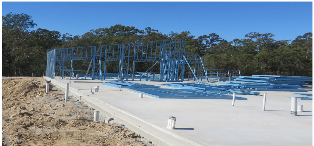
ERECTION OF WALL FRAMES
