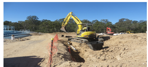
INSTALLATION OF ELECTRICAL AND COMMUNICATION SERVICES
